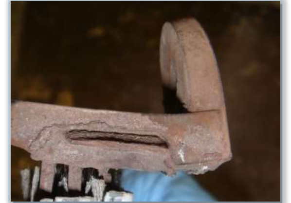
Deformation of bridge
