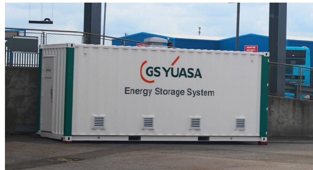
GS Yuasa Portsmouth Port Battery System
